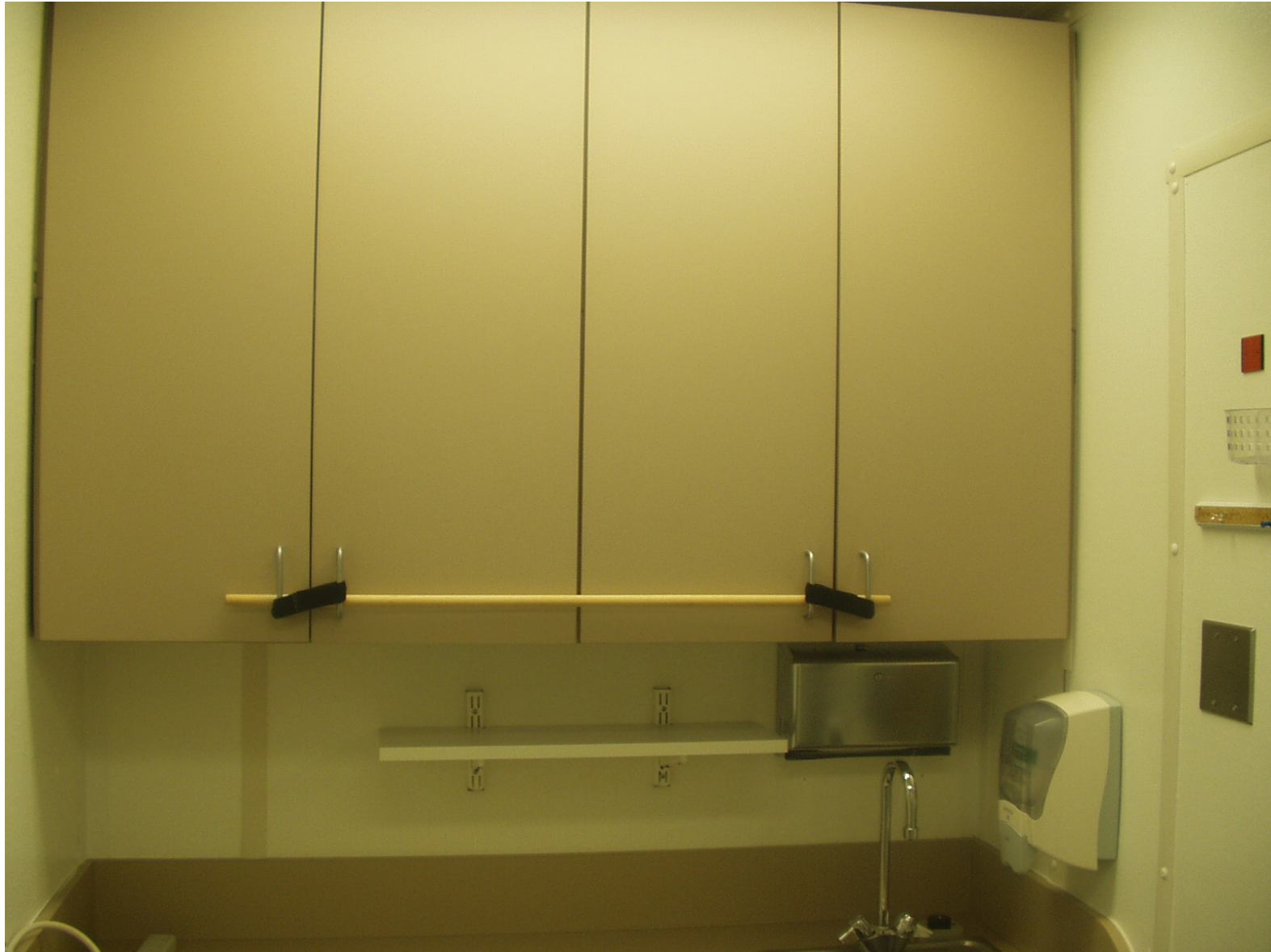
DENTAL ROOM CABINETS, SHELF AND COUNTERTOP: Remove all items from shelf above sink and countertop. Secure cabinet doors as shown with the dowel and Velcro strips.
