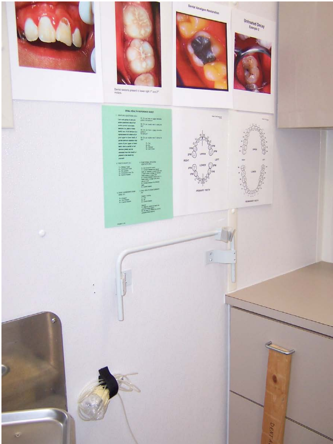
AIR SYRINGE: Air syringe wrapped in bubble wrap. Hose loosely bundled with syringe and secured to wall with Velcro strip. Reference cards remain on wall.
