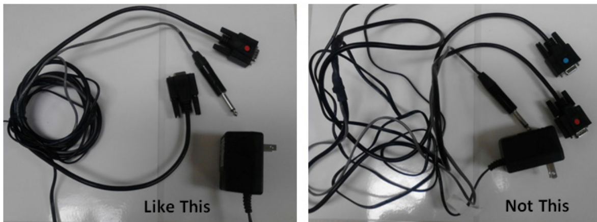
Exhibit 2-74. Correct and incorrect ways to manage extra cable length
