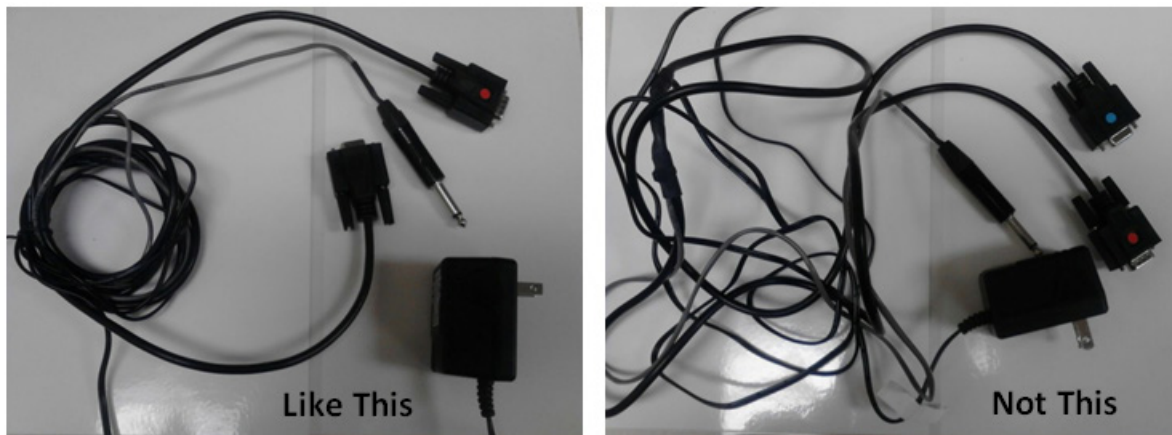
Exhibit 2-78. Correct and incorrect ways to manage extra cable length
